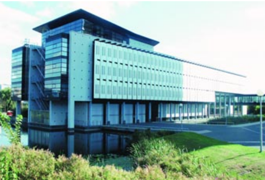
Provinciehuis op kantorenlocatie Pettelaar Park/ Provincial government building at office location Pettelaarpark
